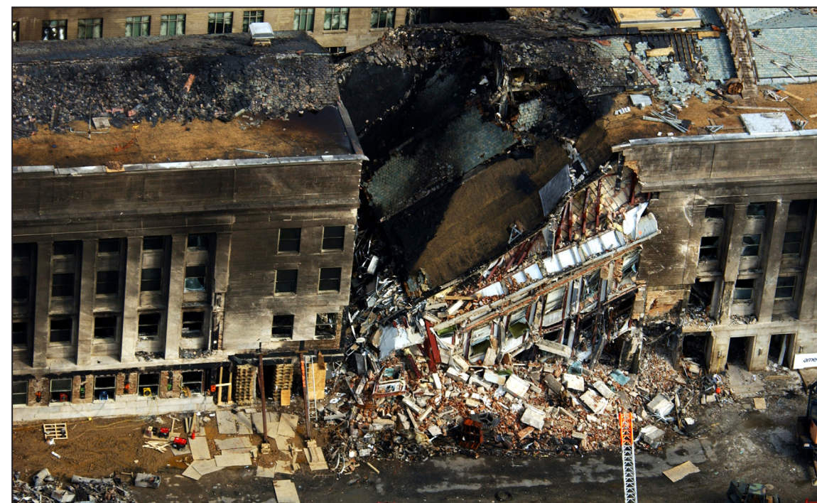
After Collapse of Central Segment
