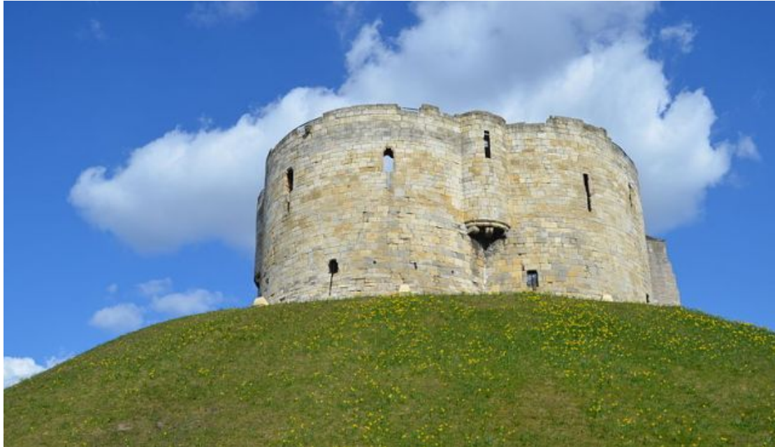
The stone structure that today stands at the site of the wooden tower where the York Massacre took place. Photo by Wikimedia Commons
