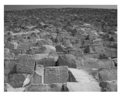
**Figure 250:** The Great Pyramid at Giza in Egypt was built thousands of years ago with 2.3 million stone blocks weighing on average between 2.5 and 15 tons.
